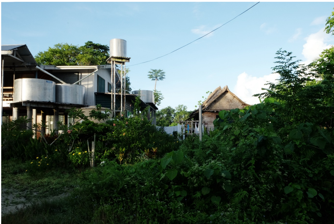
Figure 3. Rainwater catchment tanks at the Island Transit Motel. Rainwater is the only potable source of fresh water on Taro Island.
